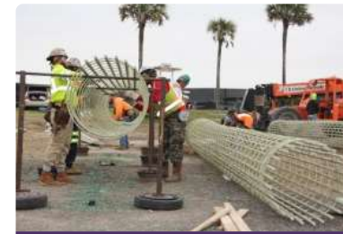
Ready to use FRP Reinforced bored piles, Florida, USA
