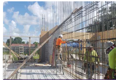
Townhouse, USA, 2019 The townhouse located in the center of Miami is fully reinforced by composite rebar
