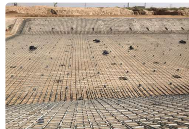
Jizan flood mitigation canal, Saudi Arabia, 2019
