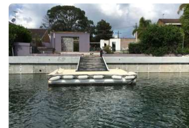
Replacement of Seawalls Slab, Australia
